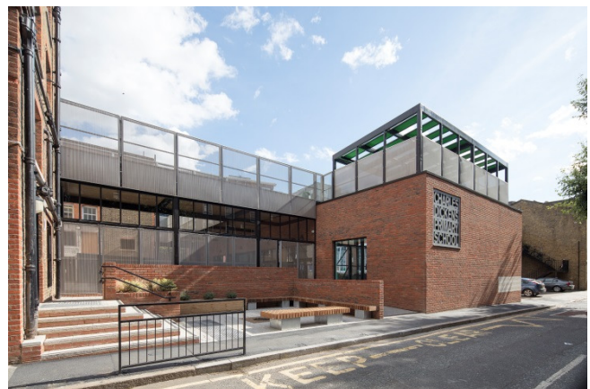
Charles Dickens School entrance incorporating old and new Haverstock Associates
