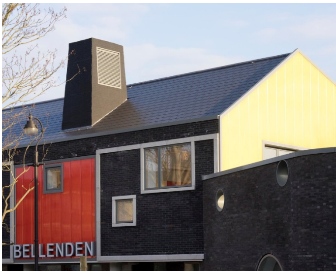
Bellenden School Cottrell & Vermeulen Architecture
